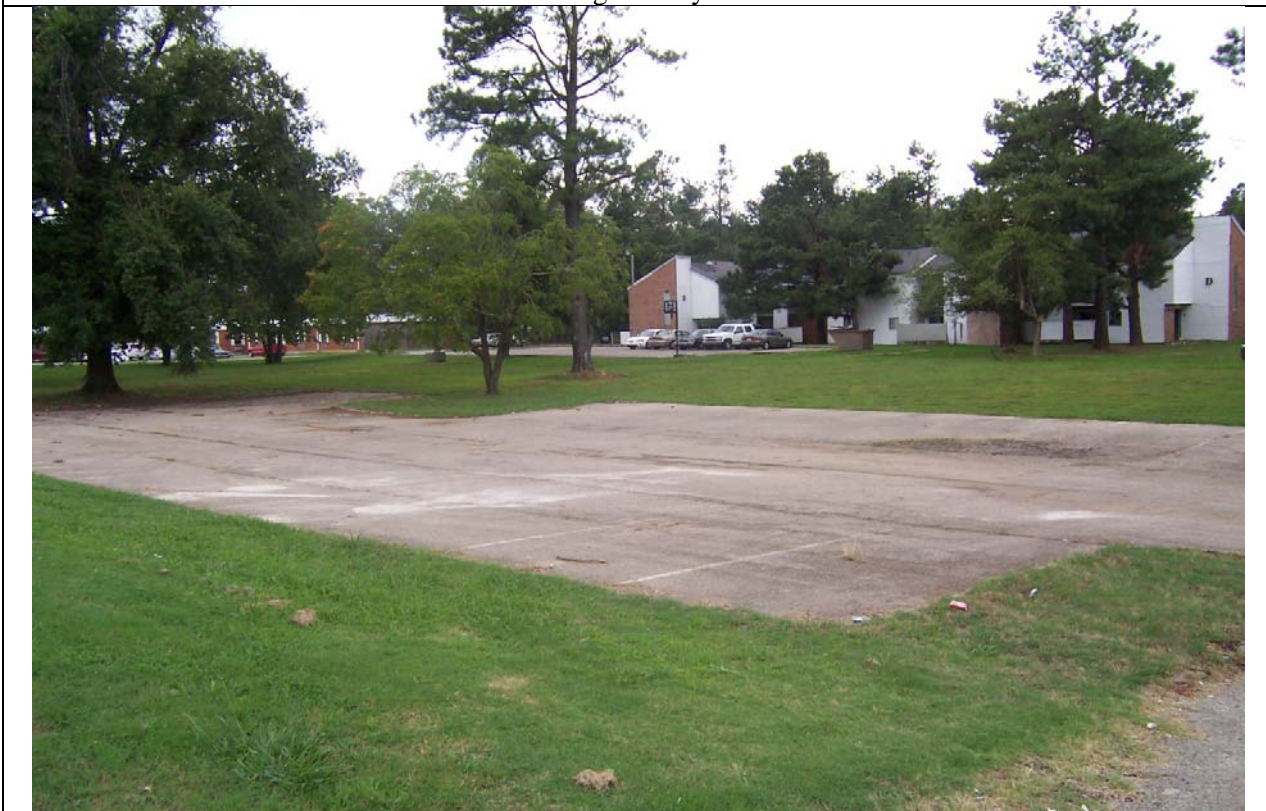
View looking northwest towards site
