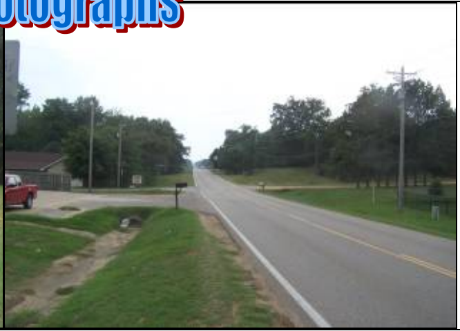
View looking South on Culberhouse
