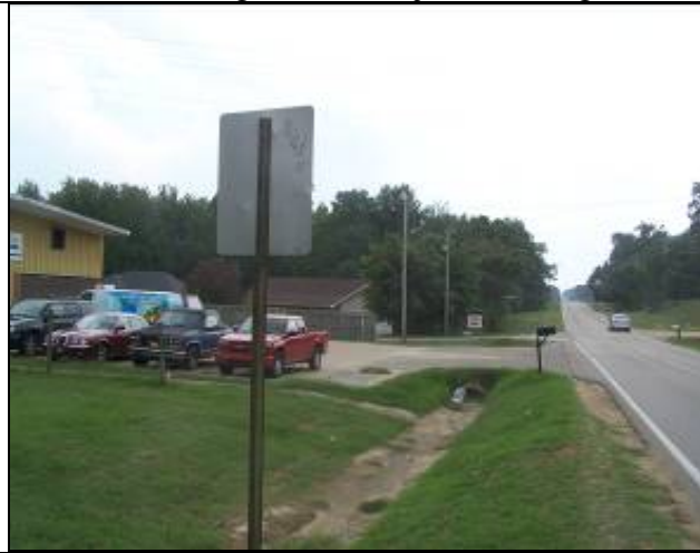
View looking North on Culberhouse
