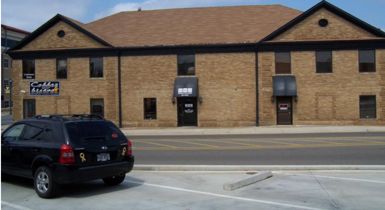
View looking at the proposed loft location.
