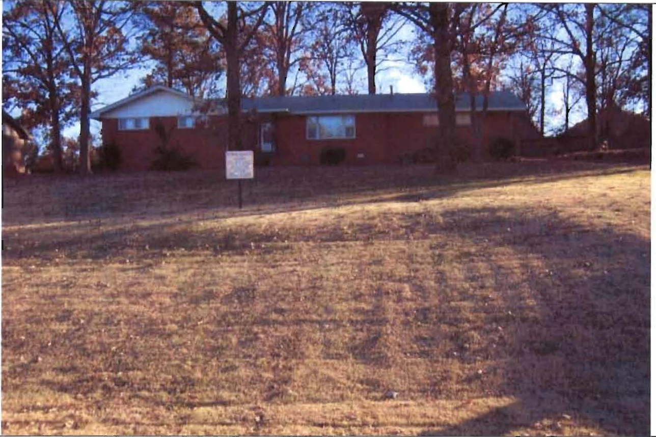
View looking south at Project Site
