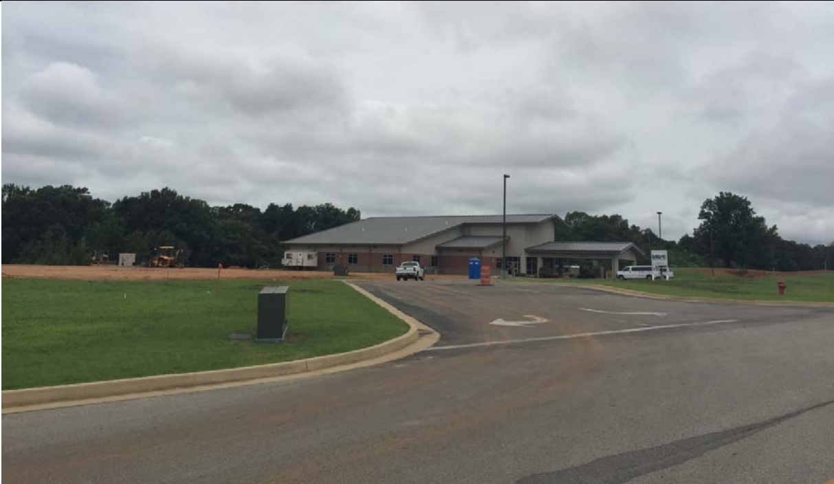
View looking Northwest from Ritter Drive towards the Forest Home Church Campus
