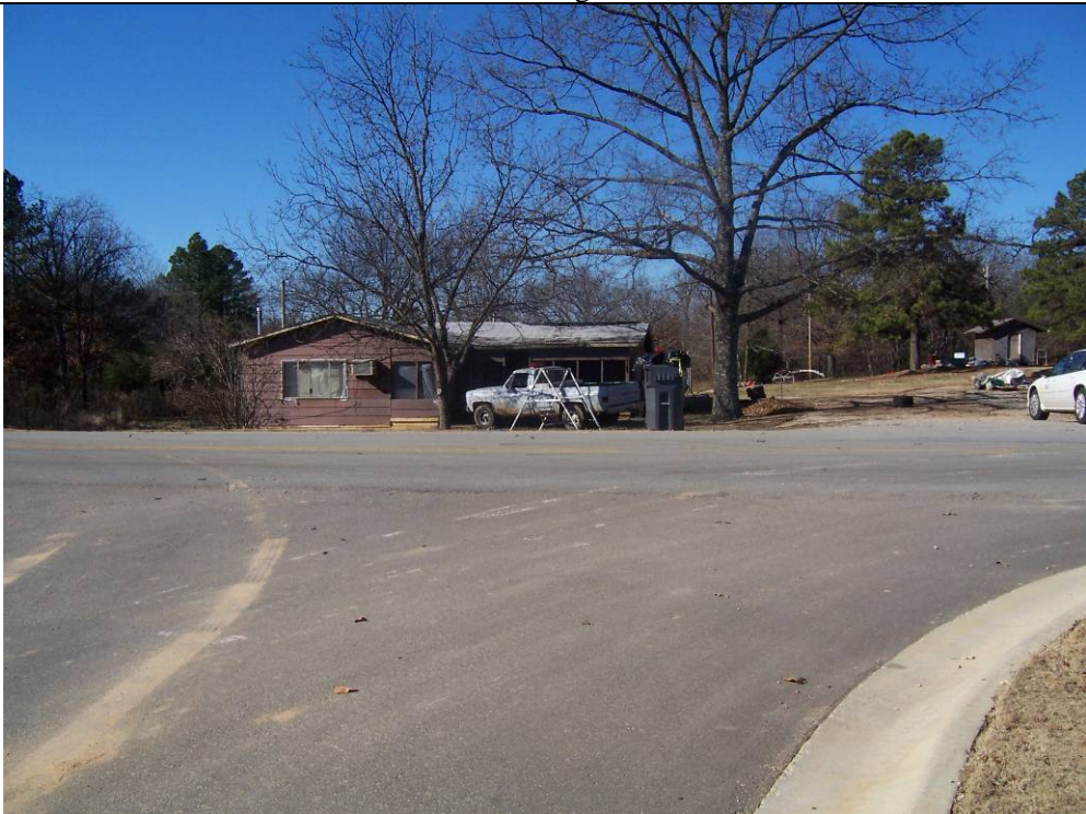
View looking at subject property looking west (former residence)
