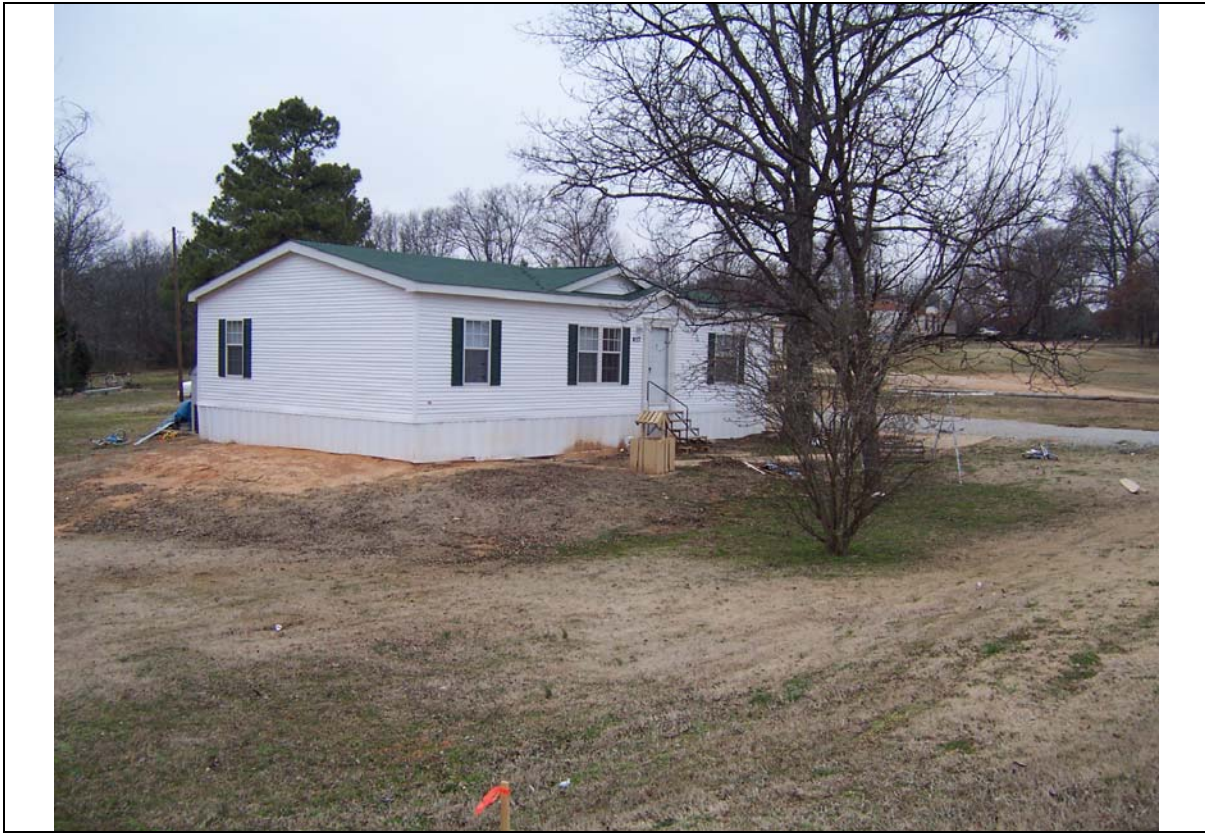
View looking west of existing unit on property frontage
