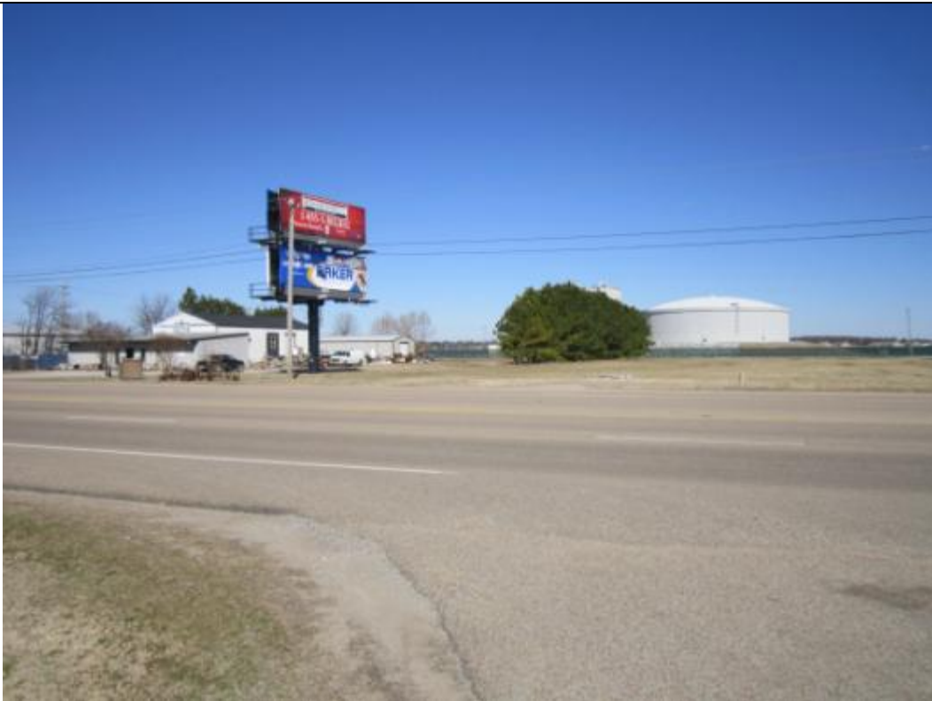
View looking northwest toward properties located to the north of subject site.
