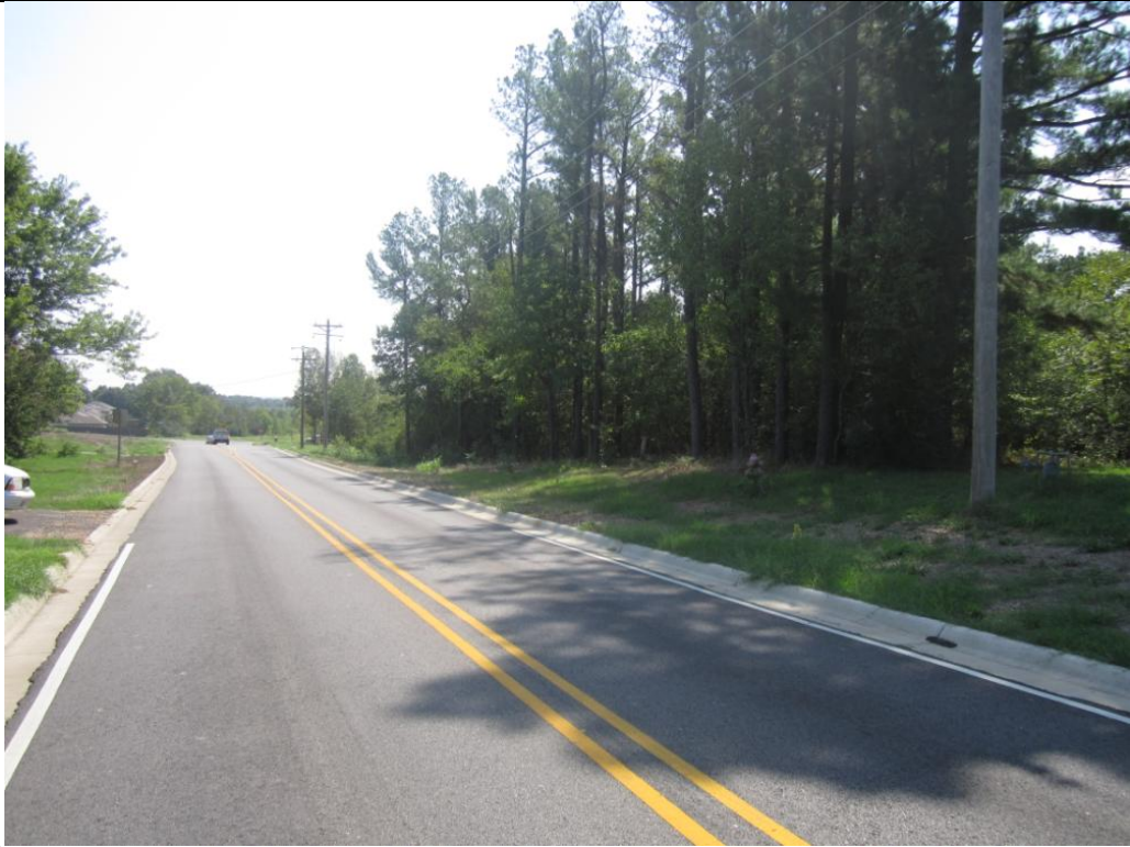
View looking East along Aggie Road
