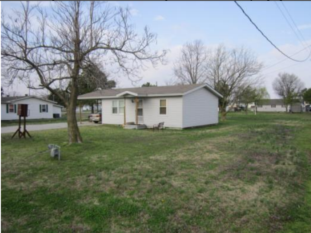
View looking southwest toward 2009 Margo Ln. One of four subject properties.
