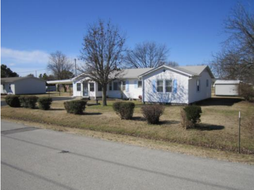
View looking southwest toward 2005 Margo Ln. One of four subject properties.
