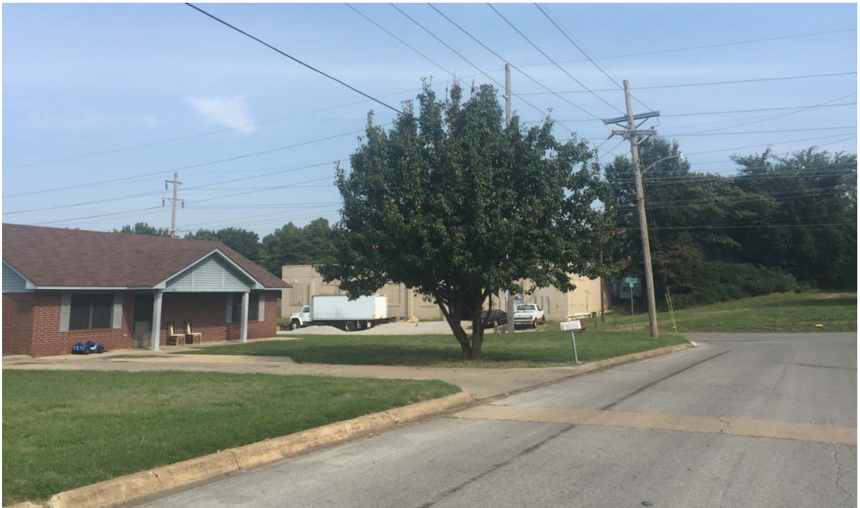
View looking north on Calion St. toward project site
