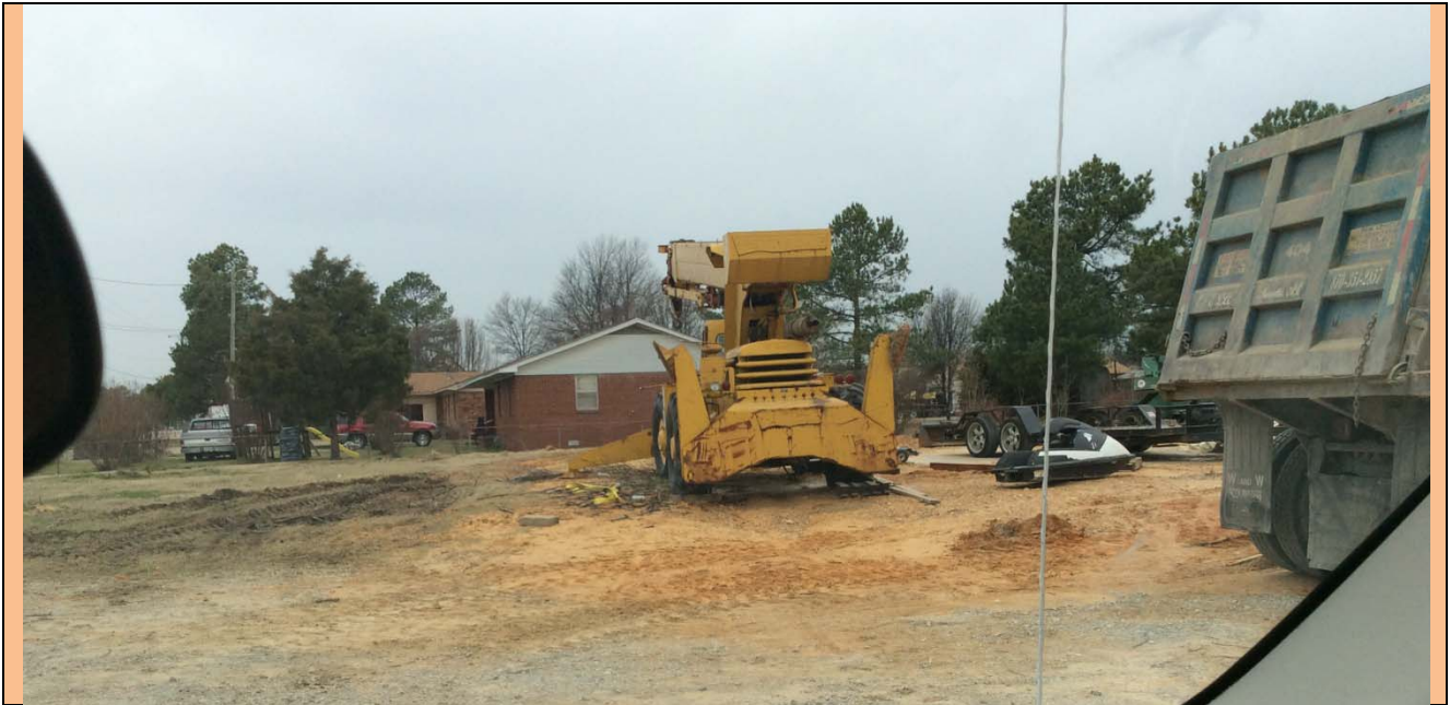
View looking West from Site
