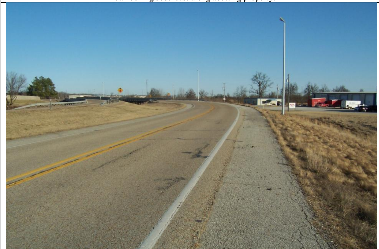
View looking southeast from subject property.
