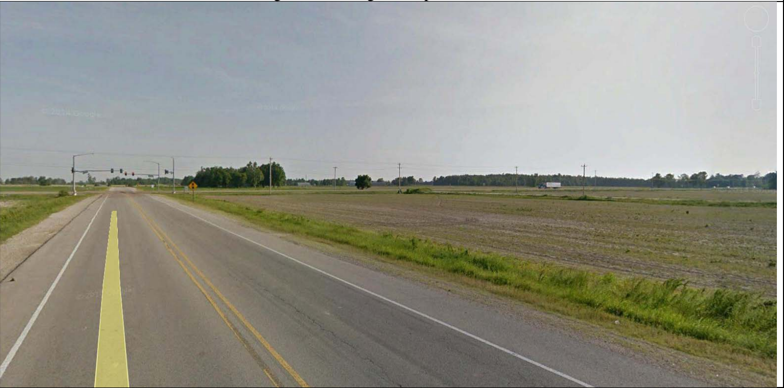
View looking South on Rogers Chapel, Site on Right
