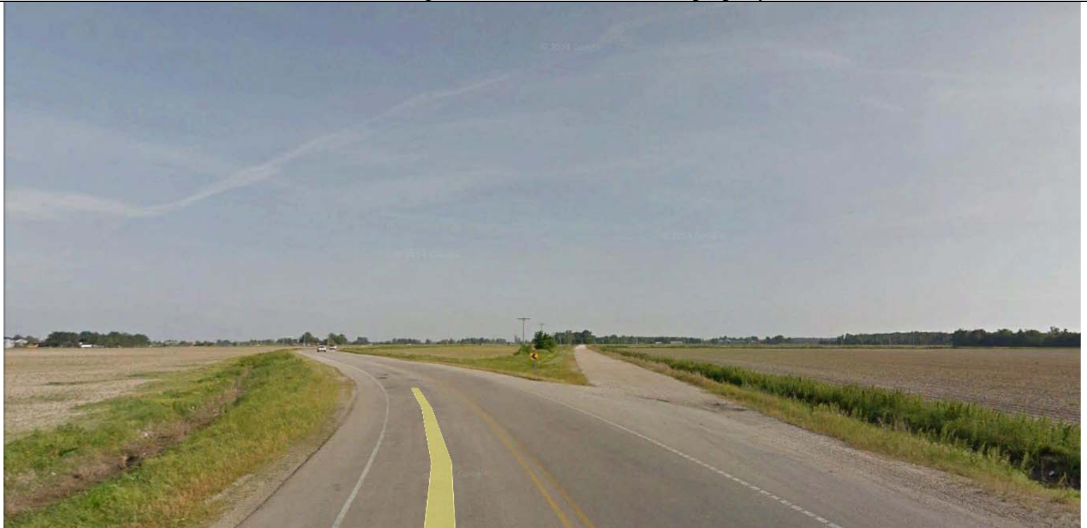
View looking South on Rogers Chapel
