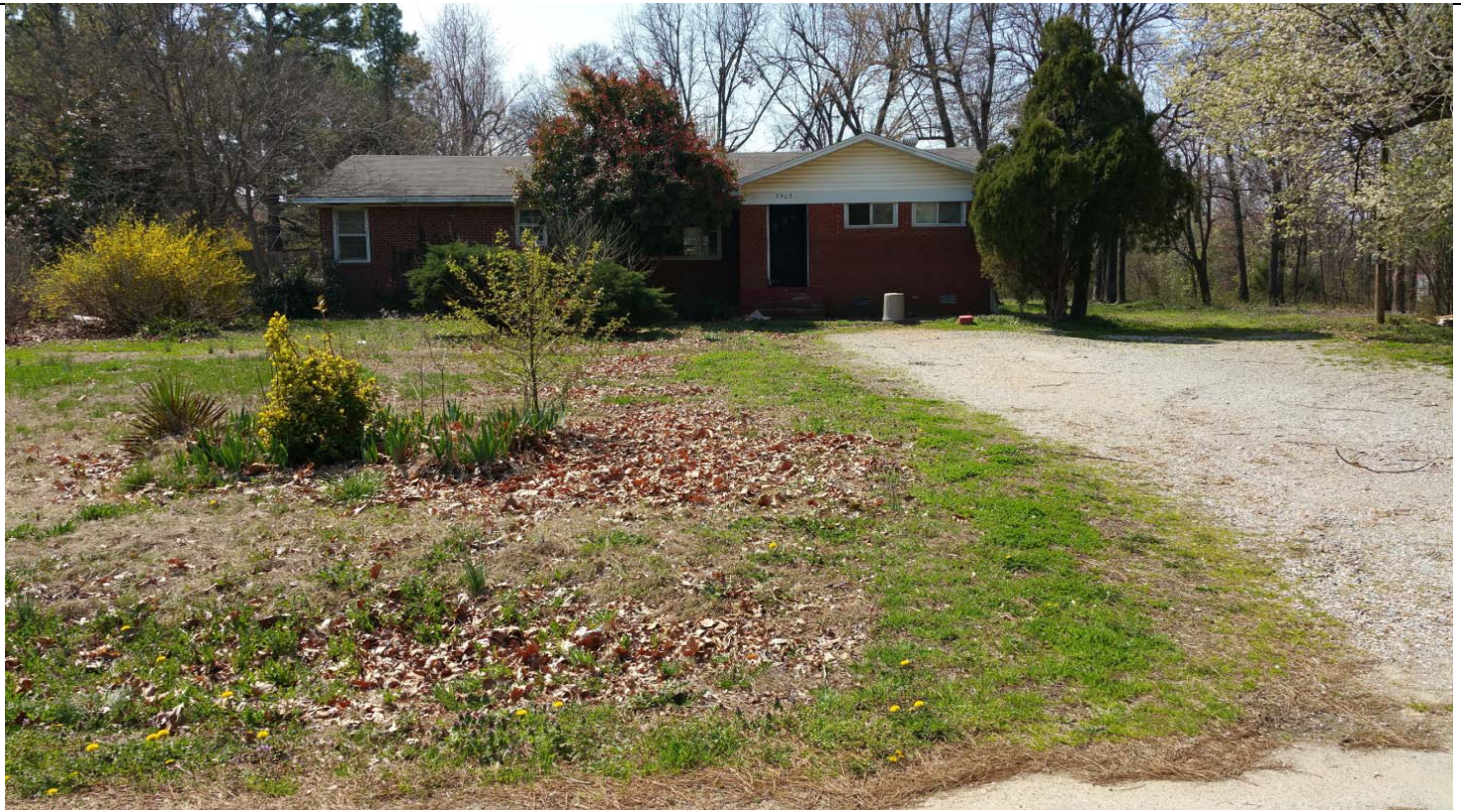
View looking at property (trailers removed)
