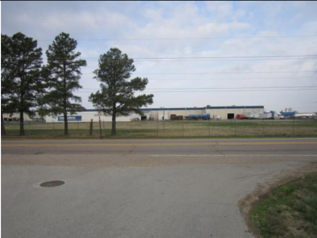
View looking west toward 5601 E. Highland Dr. which is located west of subject properties.
